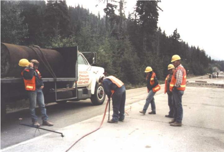
Washington Department of Transportation: Several concrete pavement sags were raised to grade by injecting grout beneath the slabs. An experienced grouting technician monitors the packer during the pressure grouting process. The packer is inserted in holes drilled in the concrete allowing the grout to be pumped under the slab. Controlled grout pressure raises the pavement to the desired grade.
