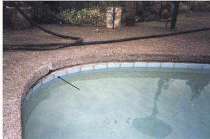
The concrete slab tilted away from the pool causing a wide gap to appear above the pool tile. The deck was successfully raised and leveled to its original elevation with a cement-pozzolan grout pumped through 1 1/2" injection pipes.
