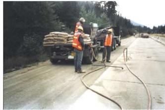
sure and any movement of the concrete slab. The grout fills voids and soft spots in the sub-surface roadbed structure without raising the concrete slabs. The cured grout provides additional supportive strength to the slab and may prevent future settling, cracks or failure of the concrete pavement.
