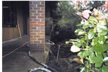
and increase load-bearing capacity of the subsoils. The walkway was leveled and brought up to proper grade with the injection of grout.
