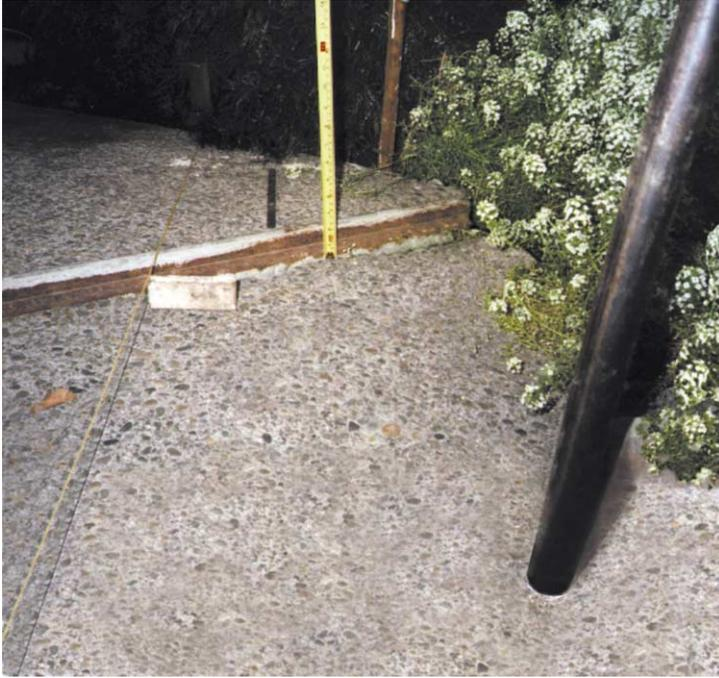
A portion of this sidewalk settled approximately 2" as evidenced by the stringline and measuring tape in the photograph above. The photo above also shows the grout packer inserted in a hole drilled in the concrete pad. Grout is pumped into the hole to fill voids under the pad. The photo at right shows additional grout pipes inserted into the ground next to the walkway. Grout is pumped into these pipes to consolidate the soils beneath the walkway
